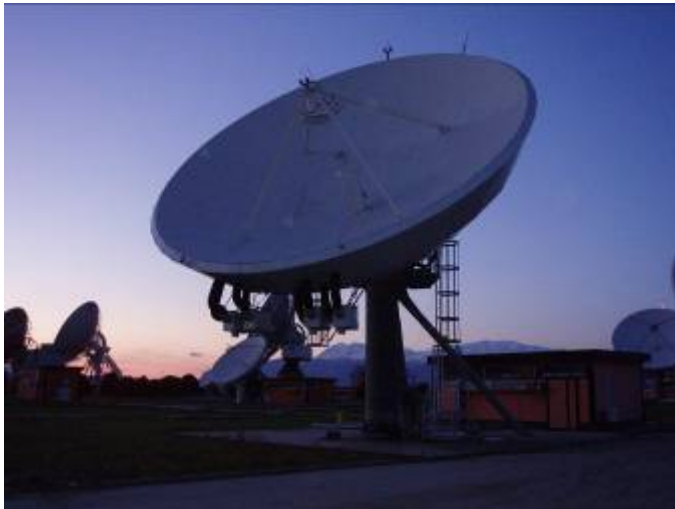
13m dish (TTC and backup)
